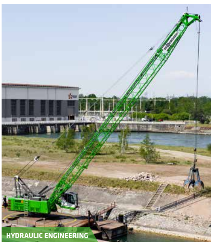
PICK & CARRY WORK WITH TELESCOPIC CRAWLER CRANES
